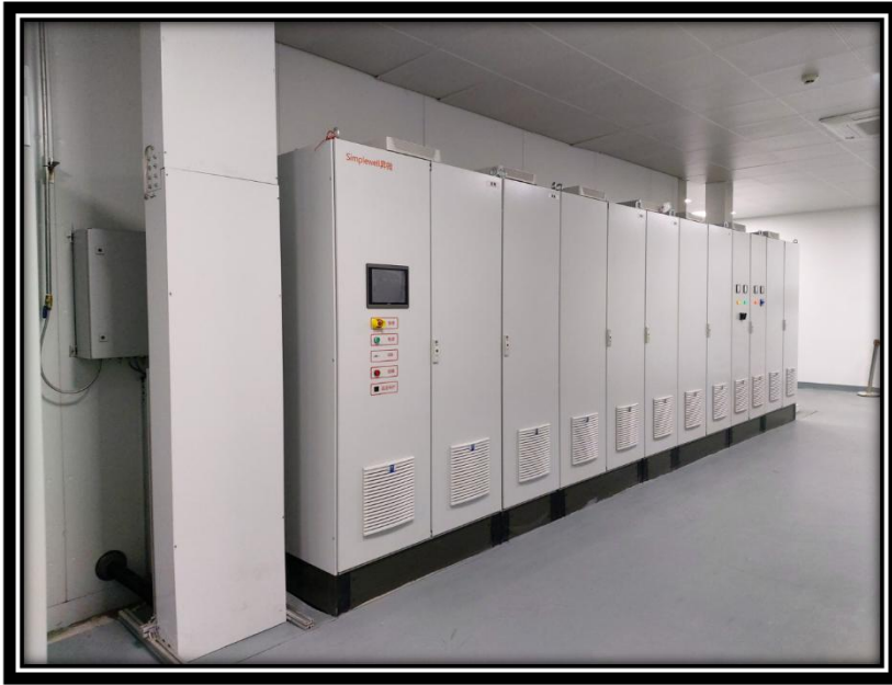
Distribution cabinet (located on the side of the freezer)
