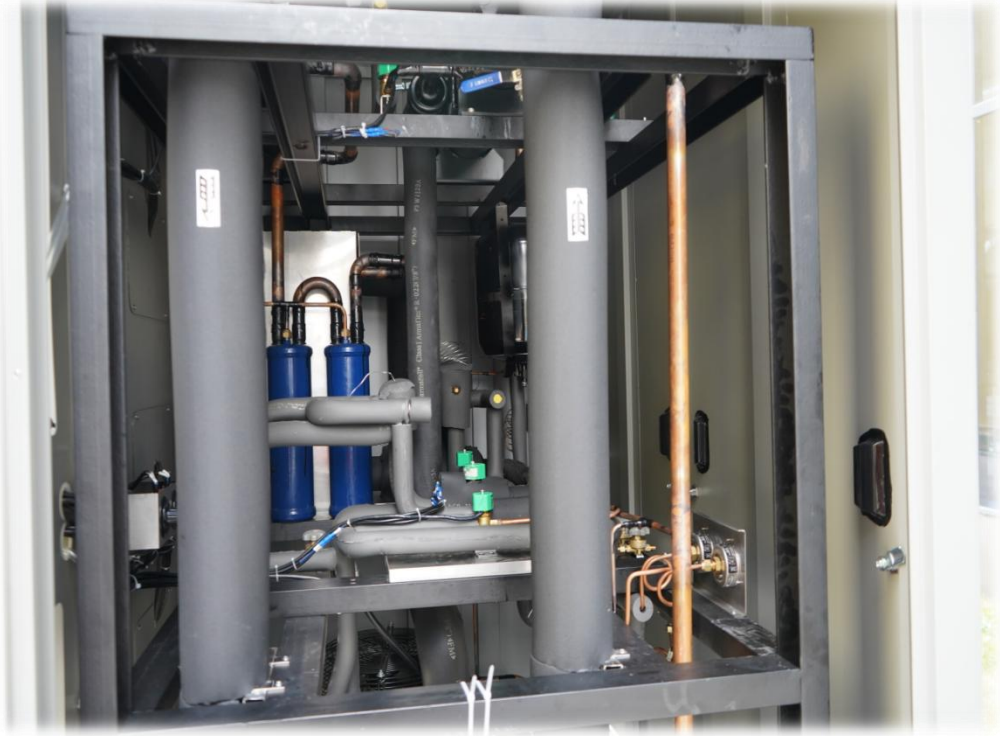
Refrigeration Unit (at the rear of the chamber)
